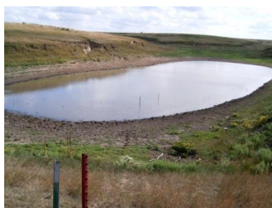
Operating Reservoir, August 2005.
